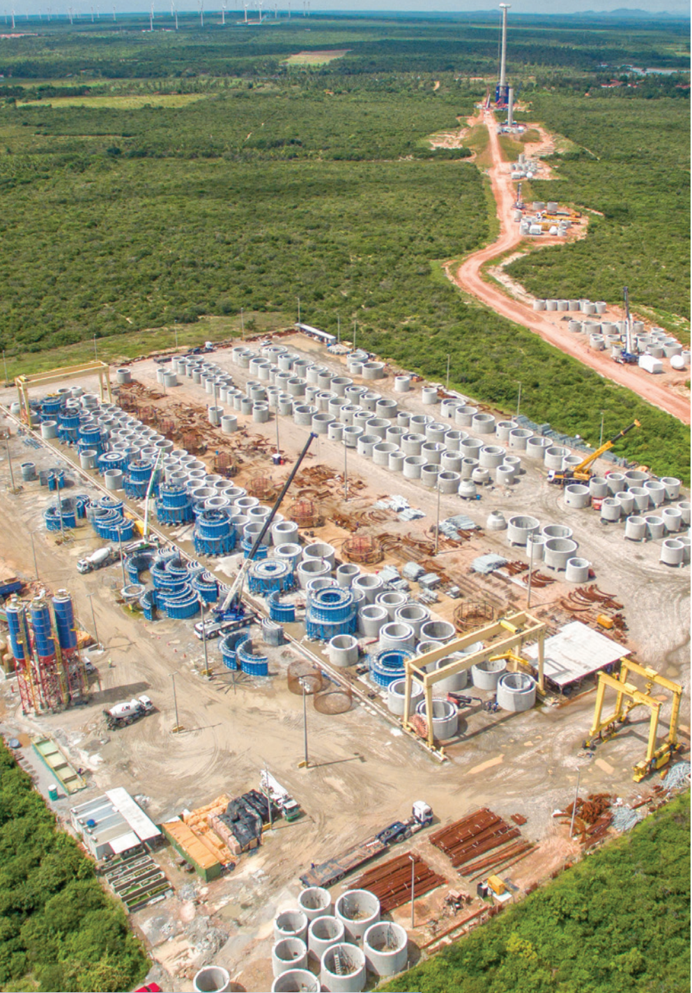
Precasting of concrete segments on site
